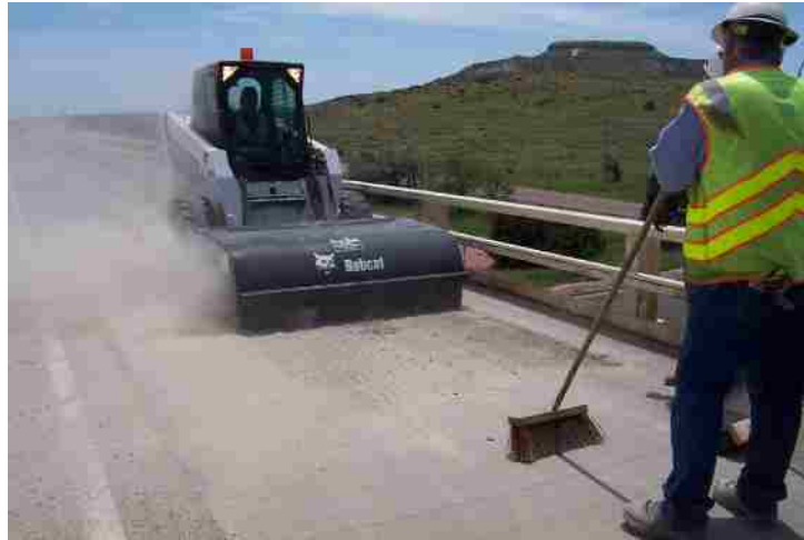
Figure 5-12 Concrete surface cleaning.
