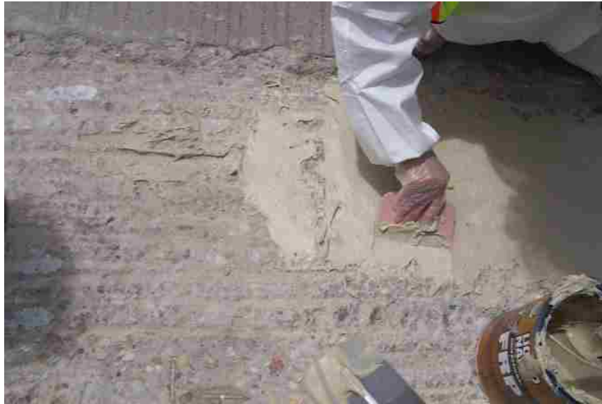
Figure 5-13 Application of putty material to obtain even concrete surface.
