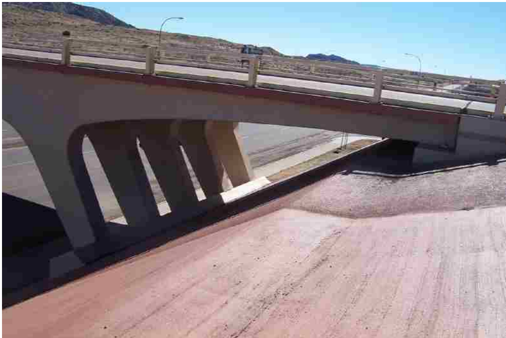
Figure 5-2 K-Frames of Bridge 7937.
