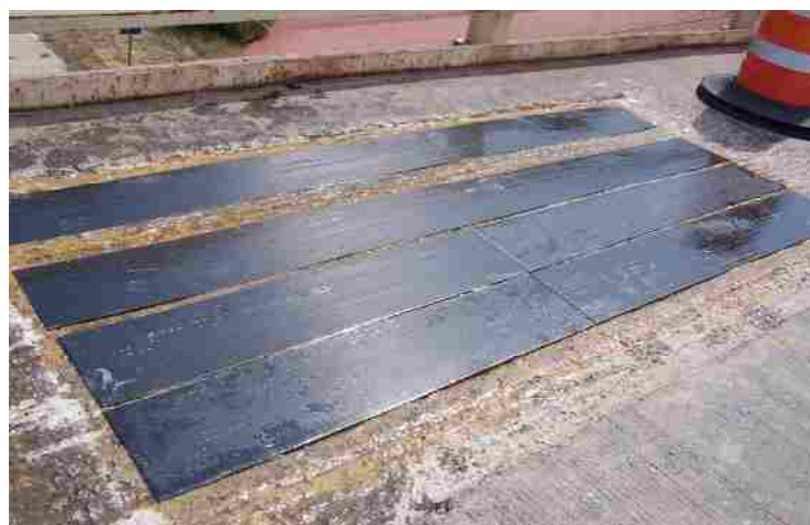
Figure 5-15 FRP strips attached to the concrete surface.
