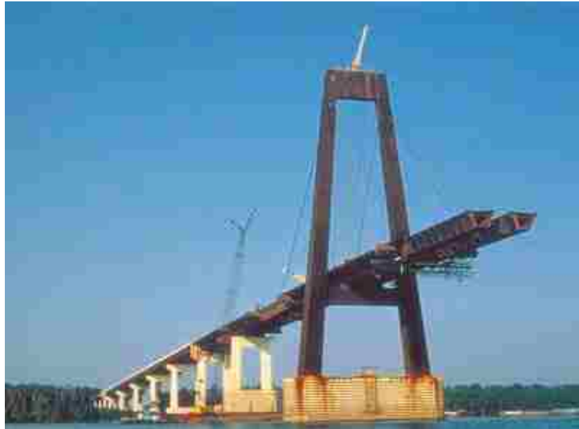
Figure 4-2 Luling Bridge during construction.
