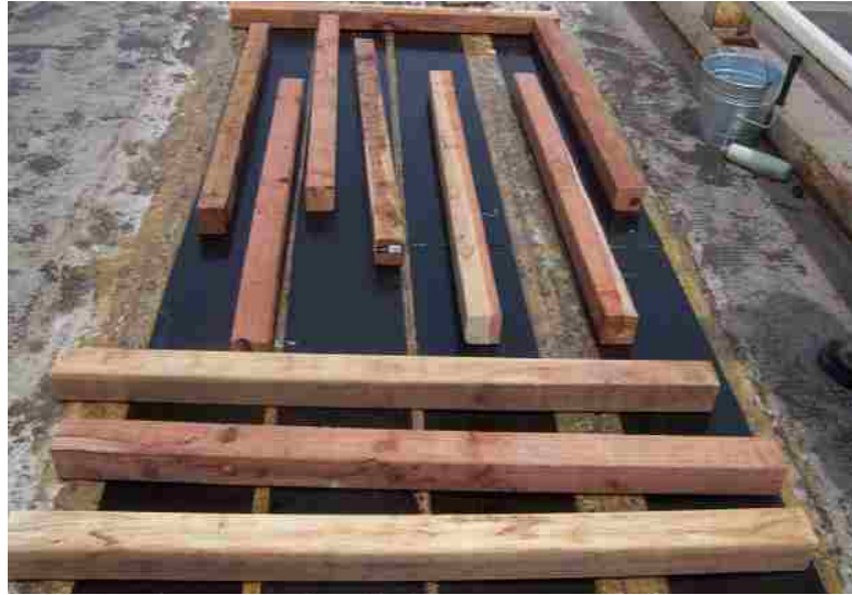
Figure 5-16 Applying pressure for better attachment of FRP strips.
